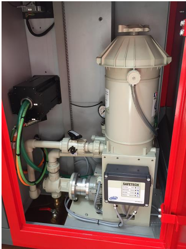
Siebec filtration device with cartridge
